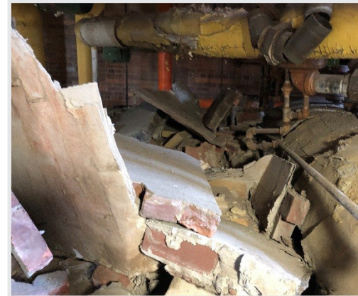
Before Photo - Top of Boiler
